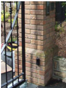
Corbelled brick pillar increasing gap size
