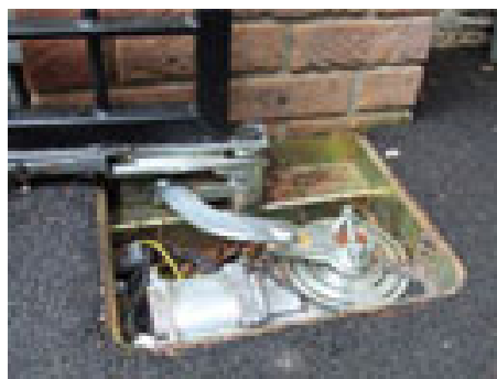
Spine of gate sat forward of mounting pin on motor, increasing gap size and creating a crushing hazard
